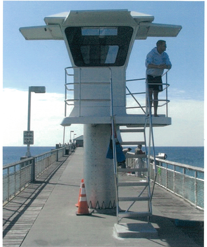
top right photo HURRICANE RESISTANT TOWER on stainless steel column. Okaloosa Pier, FL
